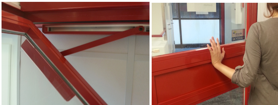
Figure 5: Weighted-closer system mounted on a door. Passing through the door will require the ability to keep it open while moving through.
